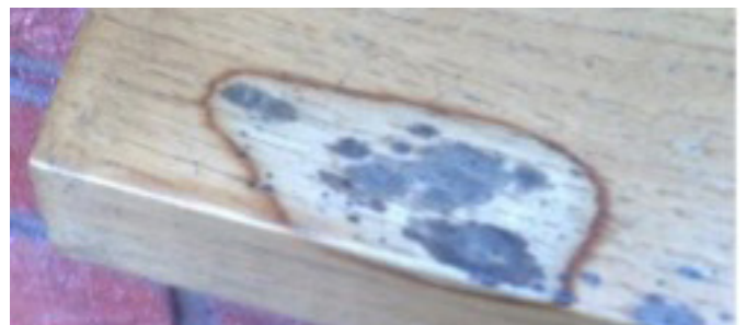
Localised staining can be sanded out using a detail sander and the coating system reinstated.
